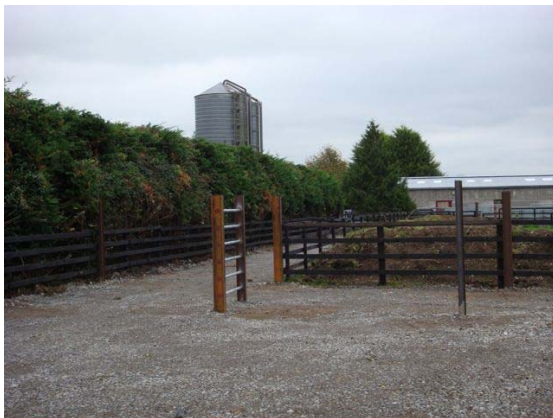
Holding pen under construction at road end of bull entrance/exit.
