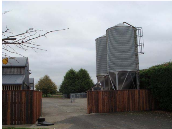
Feed bins moved nearer entrance, behind new security fence. Bin filling occurs without the feed truck entering the secure centre.
