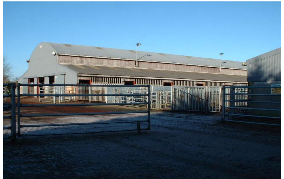
Central Performance Test Station at Tully Kildare
